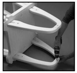
**#2:** Using two #10 x 3/4" selftapping screws, connect the Handrails together by using one screw on the outside and one screw on the inside. Repeat for the remaining handrail.
